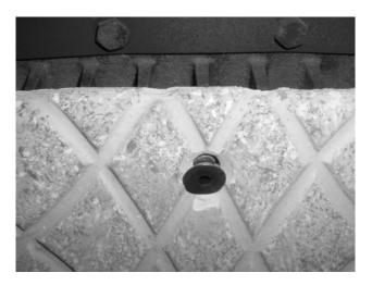
Figure 29 - Baffle Mounting Bolt
