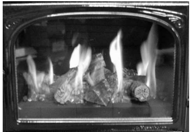
Figure 21 – Typical Burner Flame Appearance
