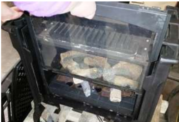
Figure 4 – Glass Removal
